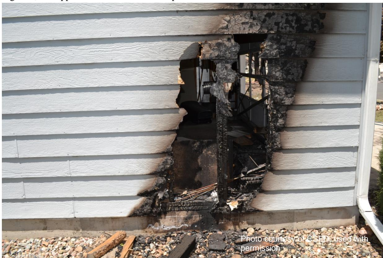
**Appendix K Figure 1** Remnants of firewood pile, which appeared to have ignited and caused ignition of the composite lap siding and thereby entry into the garage. TDs identified first responders as breaking into garage and suppressing fire.
