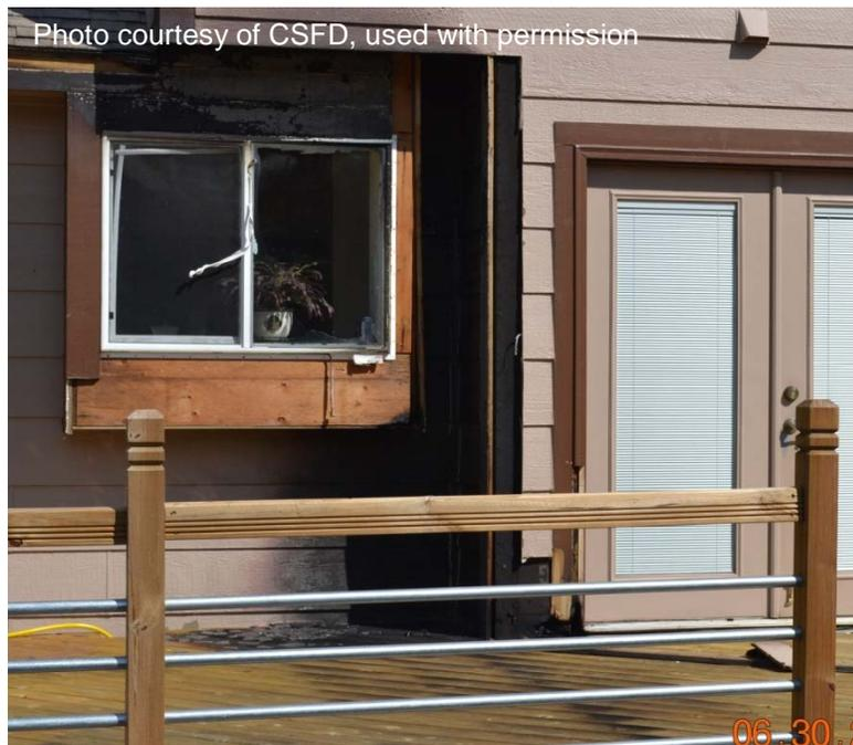
**Figure 15 Ignition in a re-entrant corner area with precise ignition location not determined in this case.**
