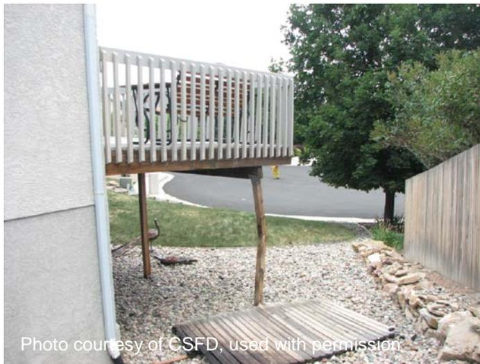
**Figure 5 Image of a burned fence piece that appeared to have broken a deck post, which had no sign of fire damage.**
