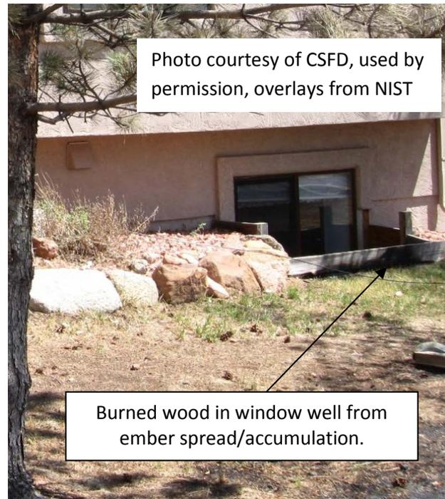
**Figure 51 Damage to wooden window well. Note the damage was not from continuous fire spread as evidenced by the green vegetation.**
