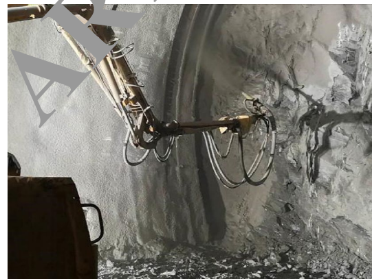
Figure. 10 Xiangshuwan No. 2 inclined shaft test's construction site
